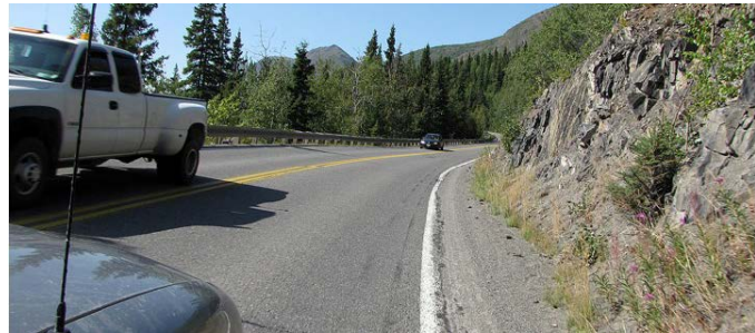
Sharp curves and narrow shoulders slow traffic and reduce visibility around corners
