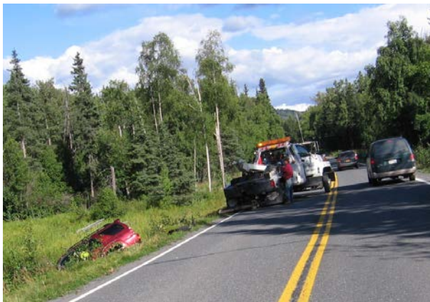
Narrow or nonexistent shoulders increase the chance for run-off-the-road crashes.
