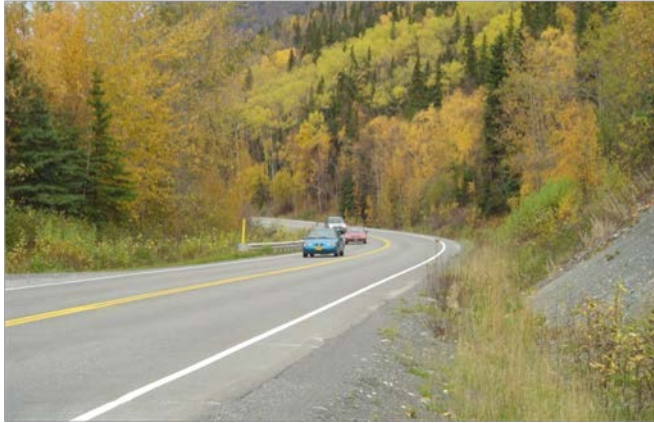
The Sterling Highway MP 45–60 area currently is characterized by sharp curves and narrow shoulders.
