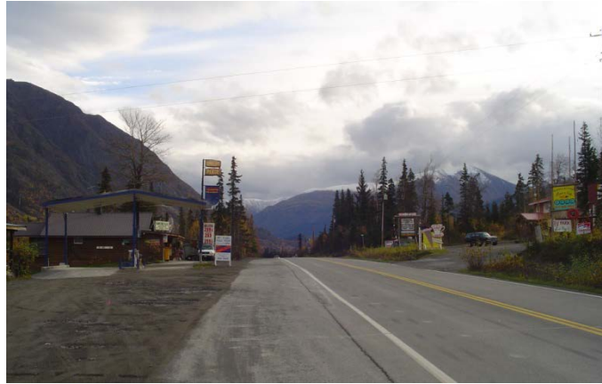
Driveways cause conflict points that slow traffic and increase the chance of crashes.
