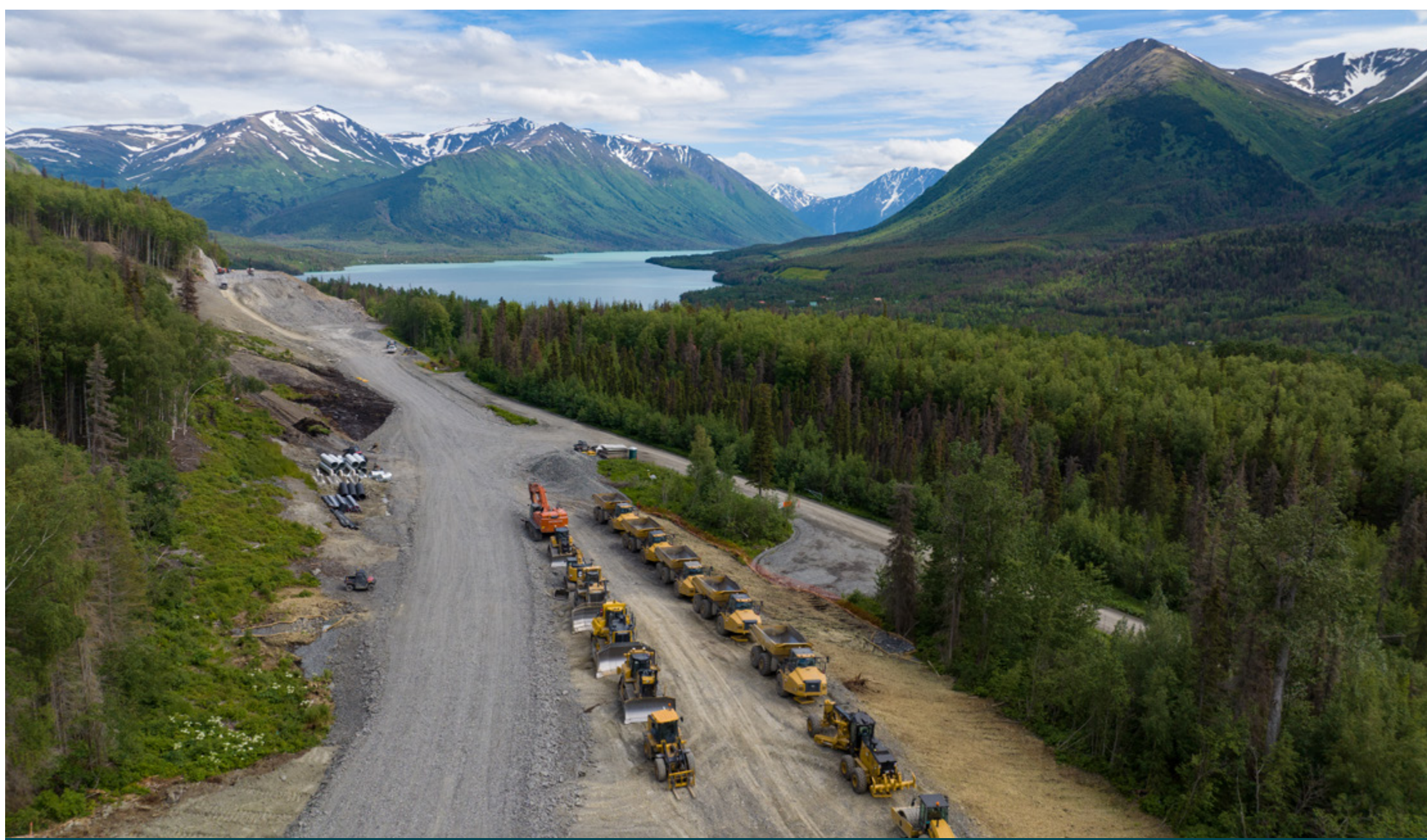
Mobilized Equipment to Phase 3 (July 2023)
