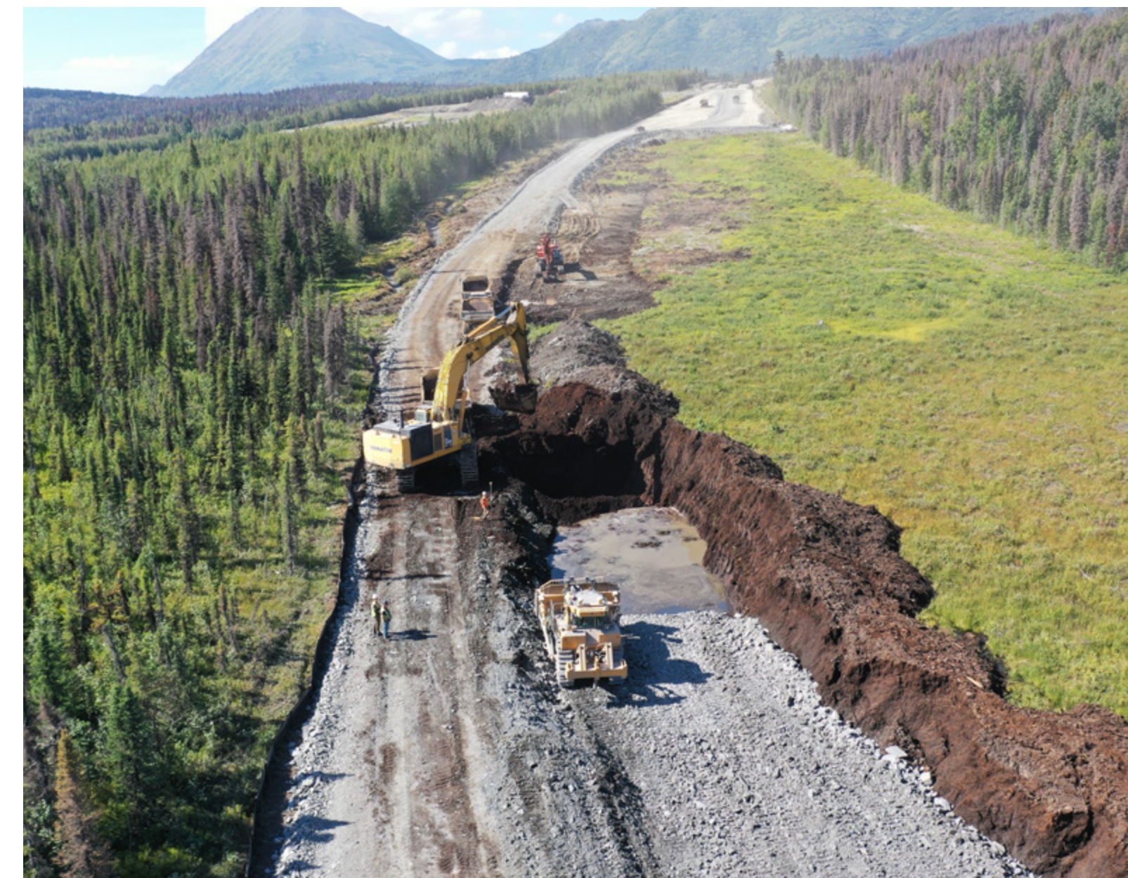
Phase 3: Equipment working in the muck excavation zone
