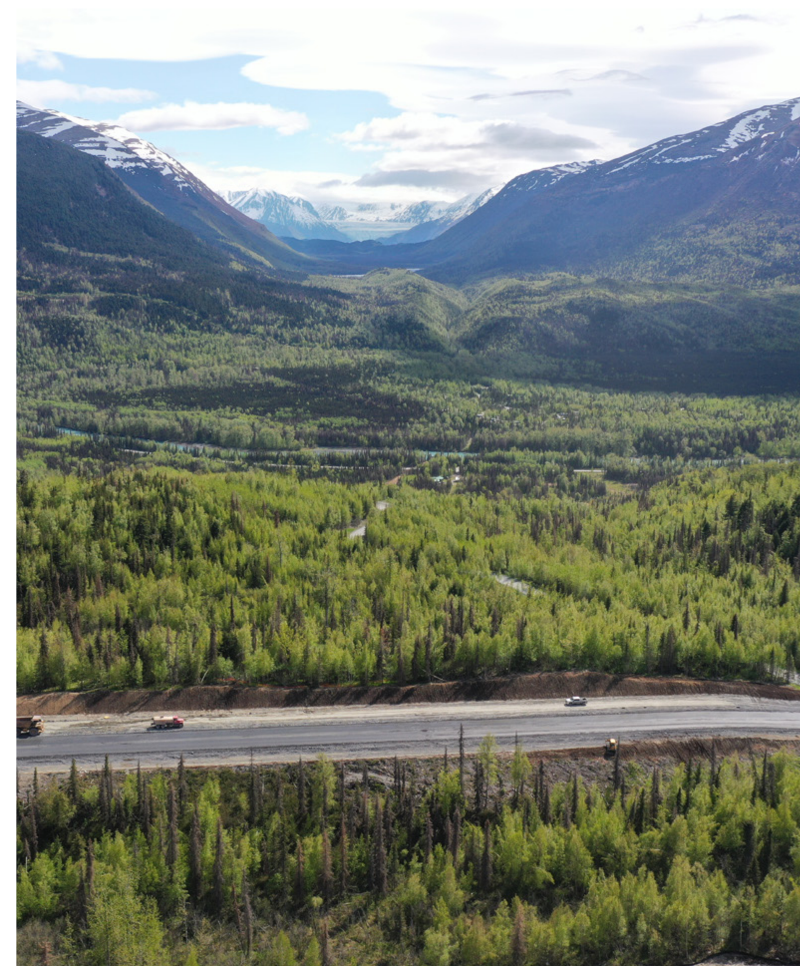
Phase 4: Location of the on and off ramp within parcel 395 with Skilak Glacier in the background.
