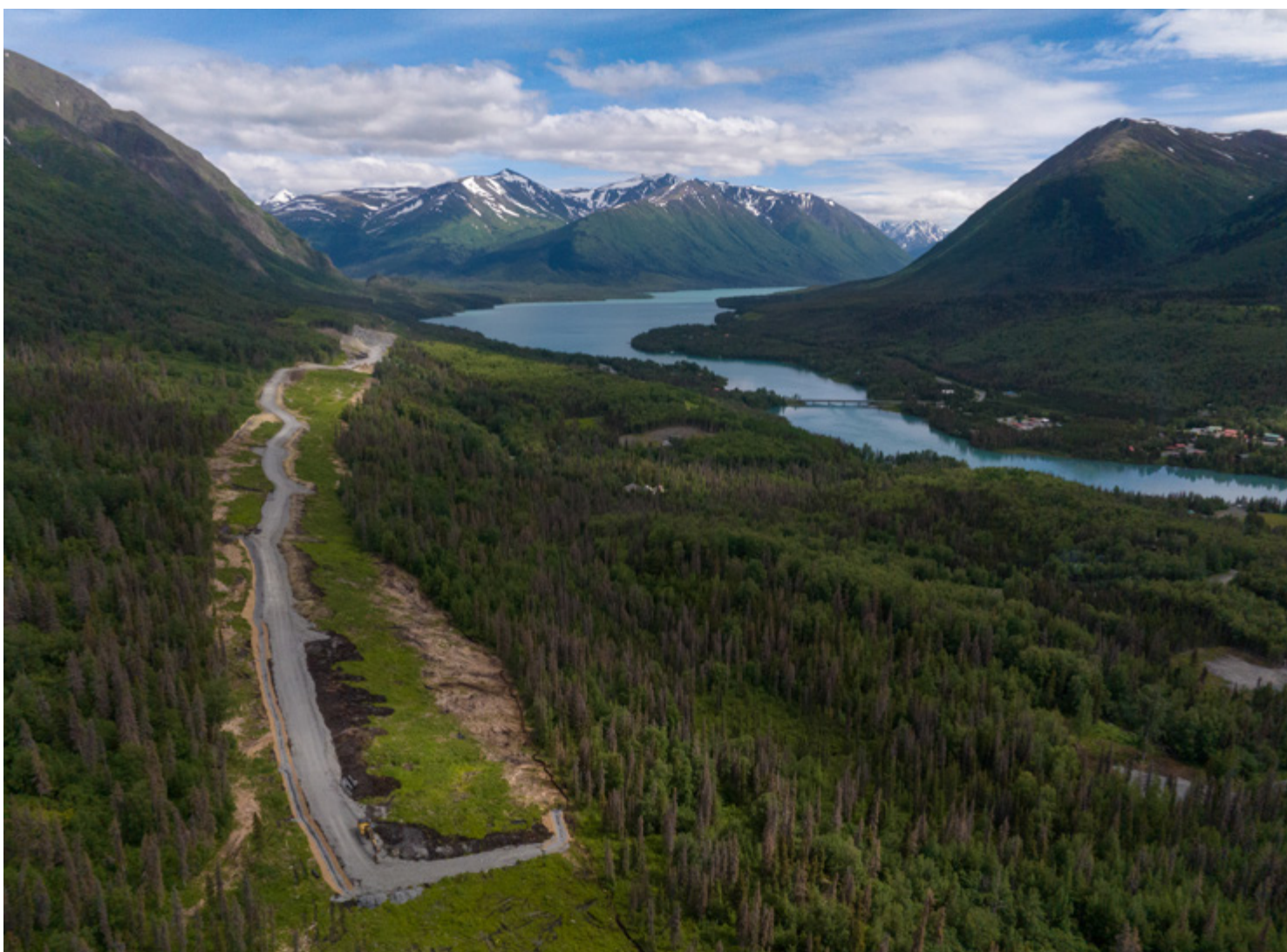
Access Road Construction to East Abutment (2023 - 2024)
