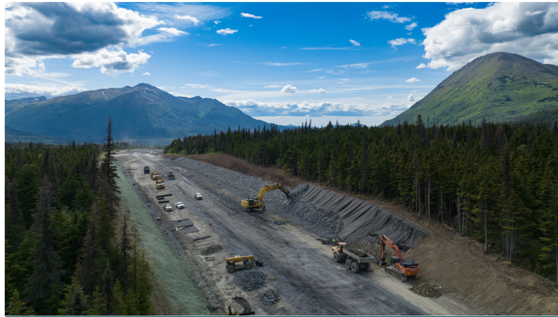
Finishing Slopes with Rip Rap and Final Stabilization
