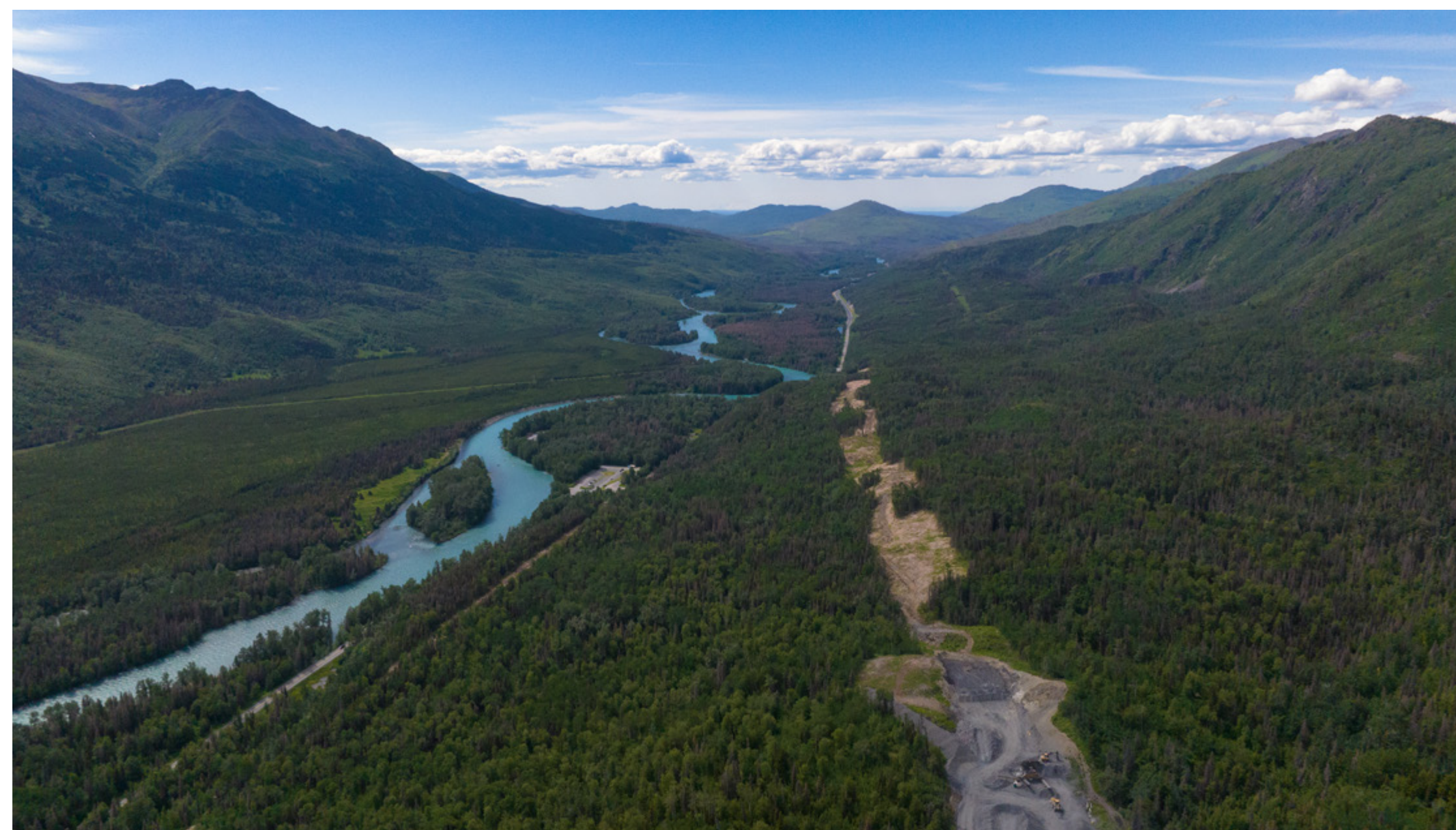
Phase 4 meets Phase 5 Clearing
