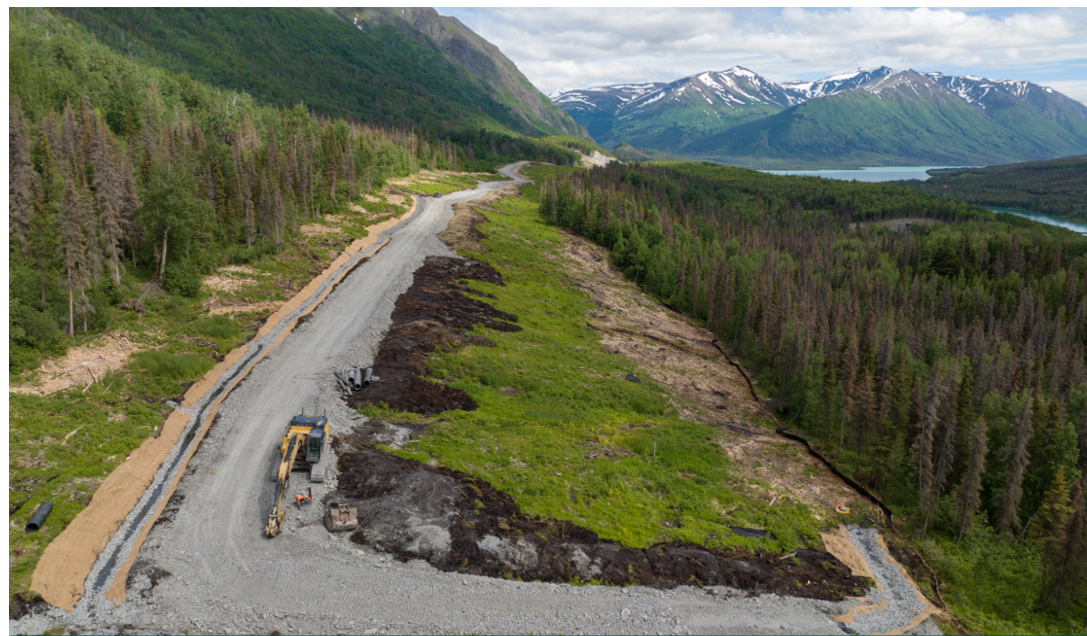
Rock Excavation and Road Construction to East Abutment
