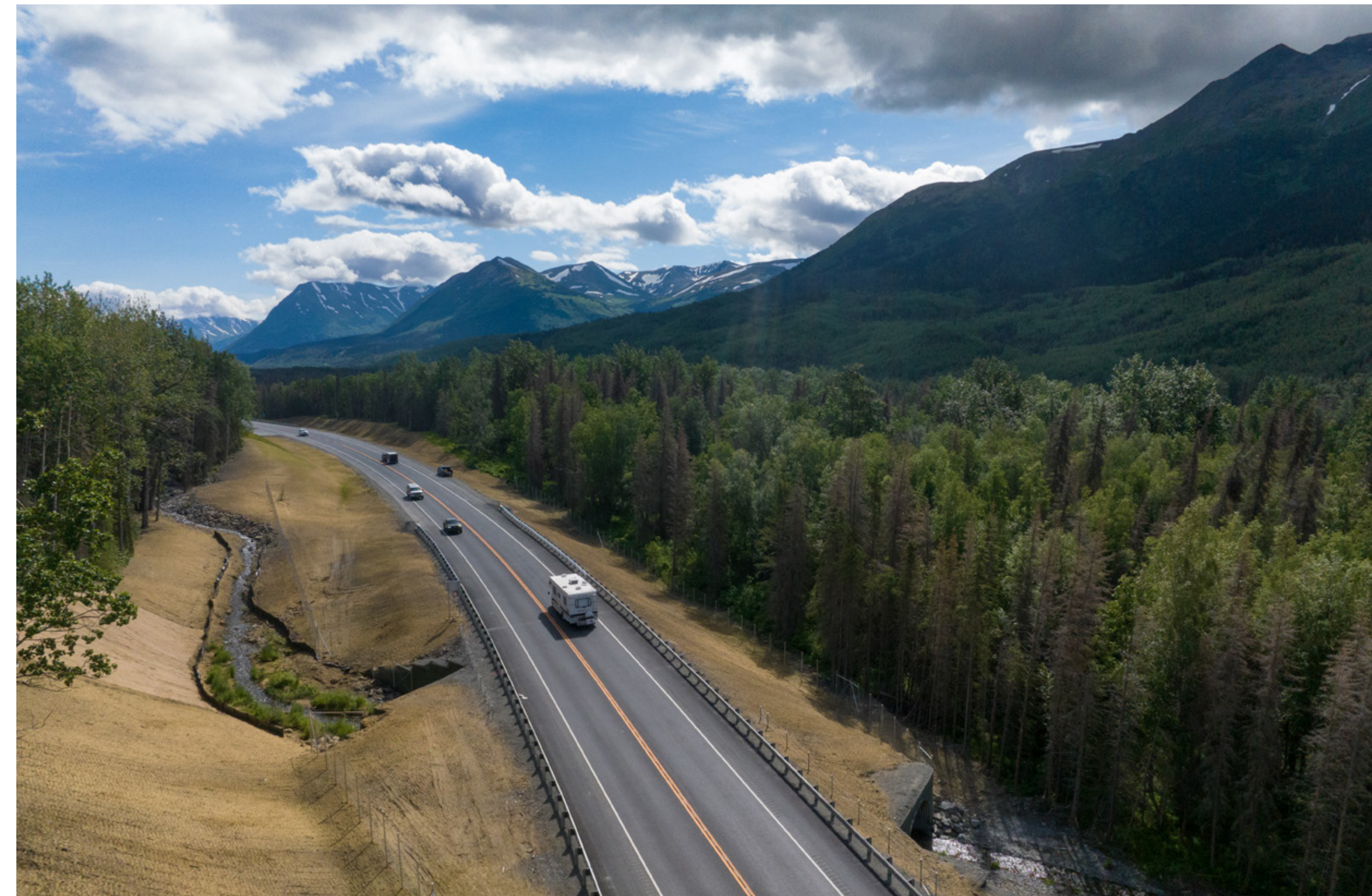
Newly completed Sterling Highway with Fuller Creek stream realignment.
