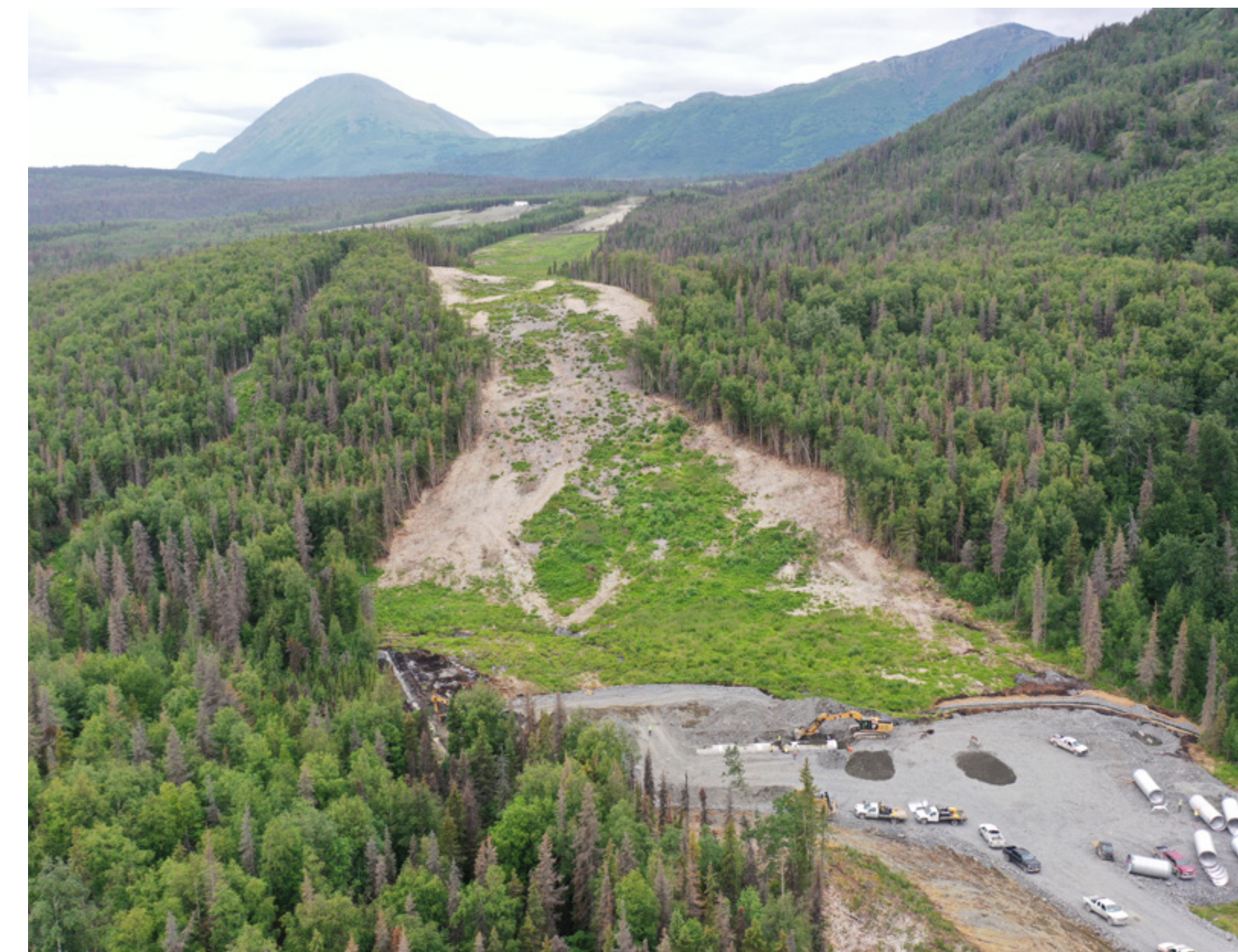
Phase 3: Fish pipe installation
