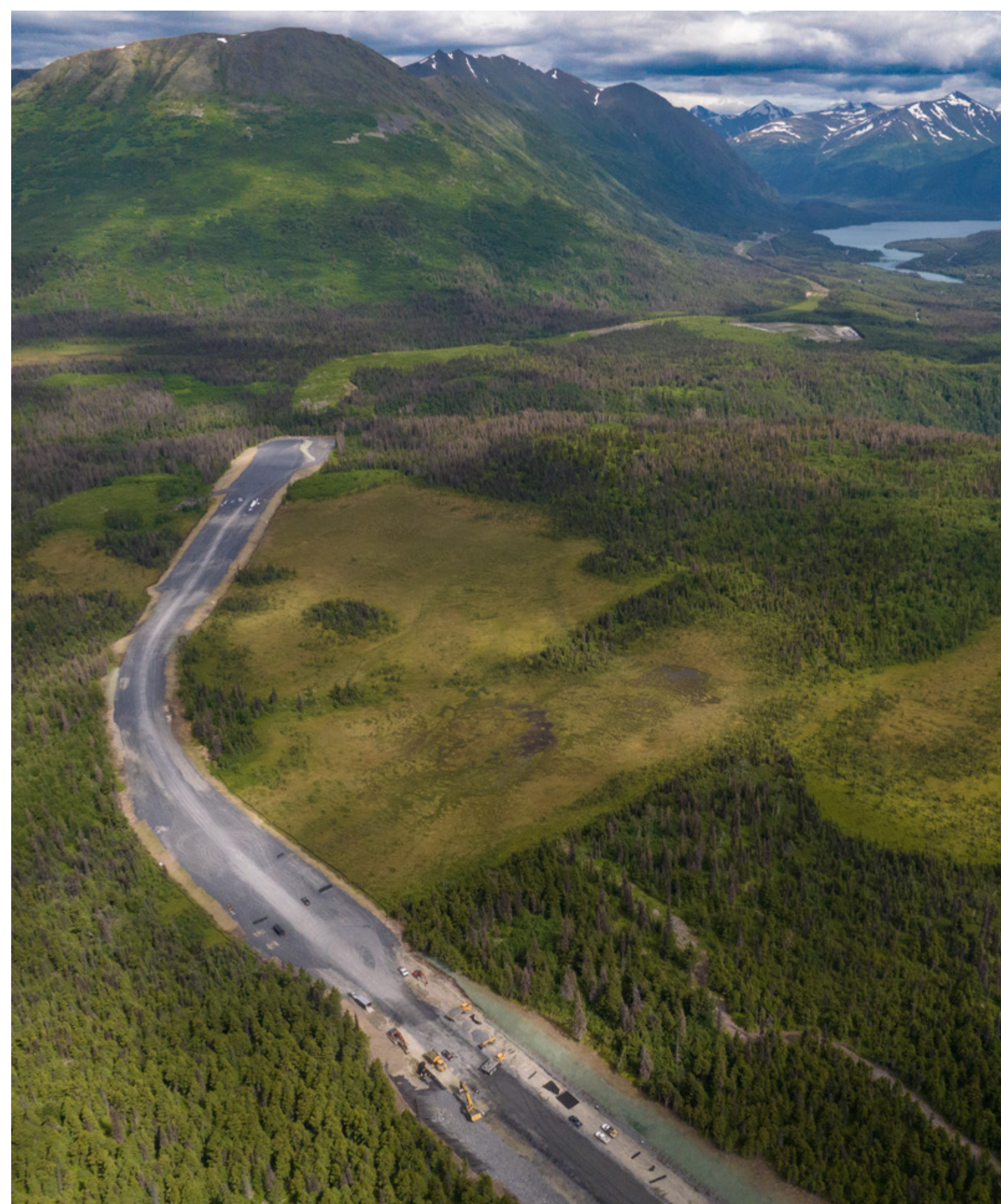
Phase 4: Constructing access to the West Bridge Abutment
