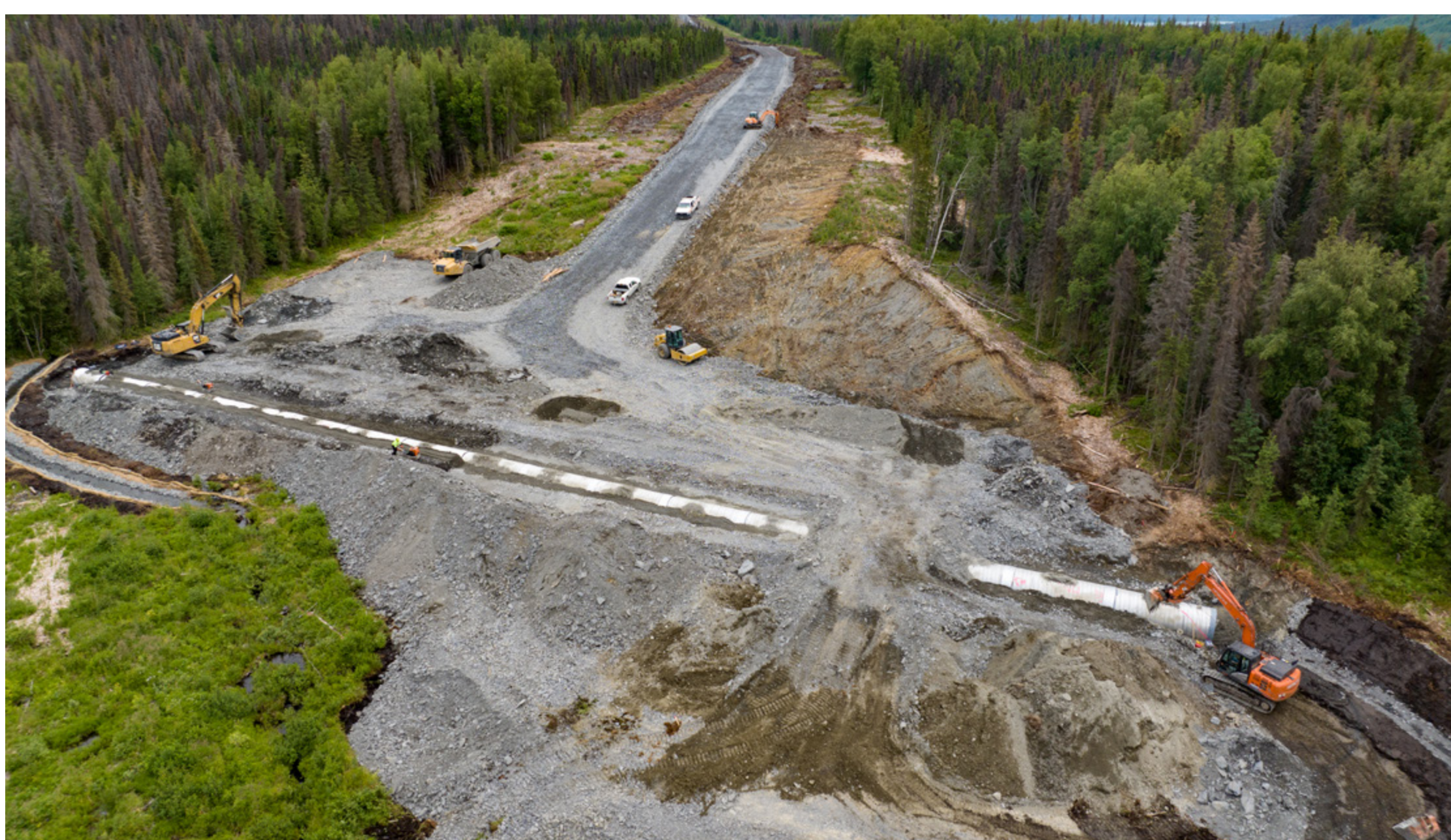
Installation of Drainage Culverts
