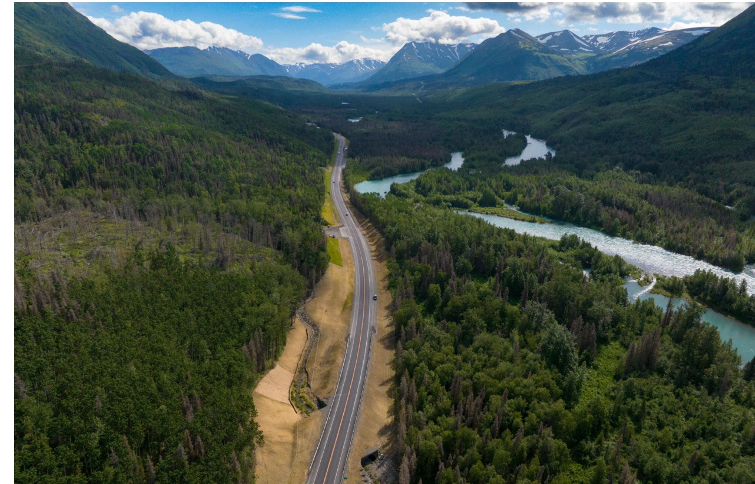
Looking east along the newly completed Sterling Highway Phase 1A.
