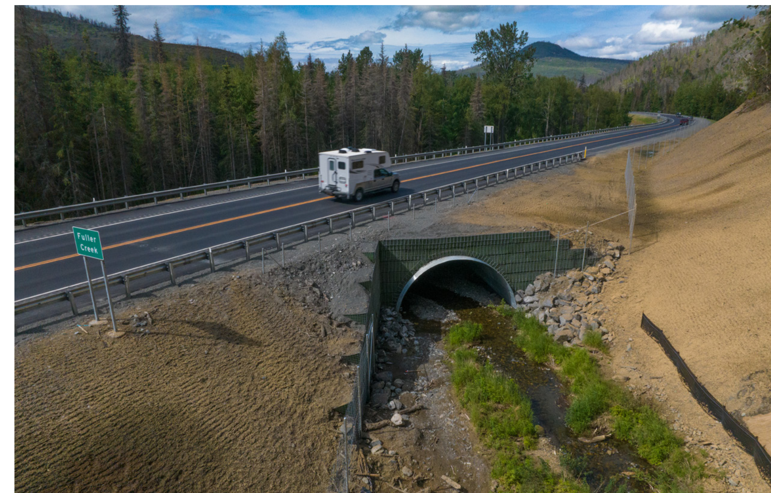
Inlet of Fuller Creek Wildlife and Fish Passage Crossing with wildlife fencing.
