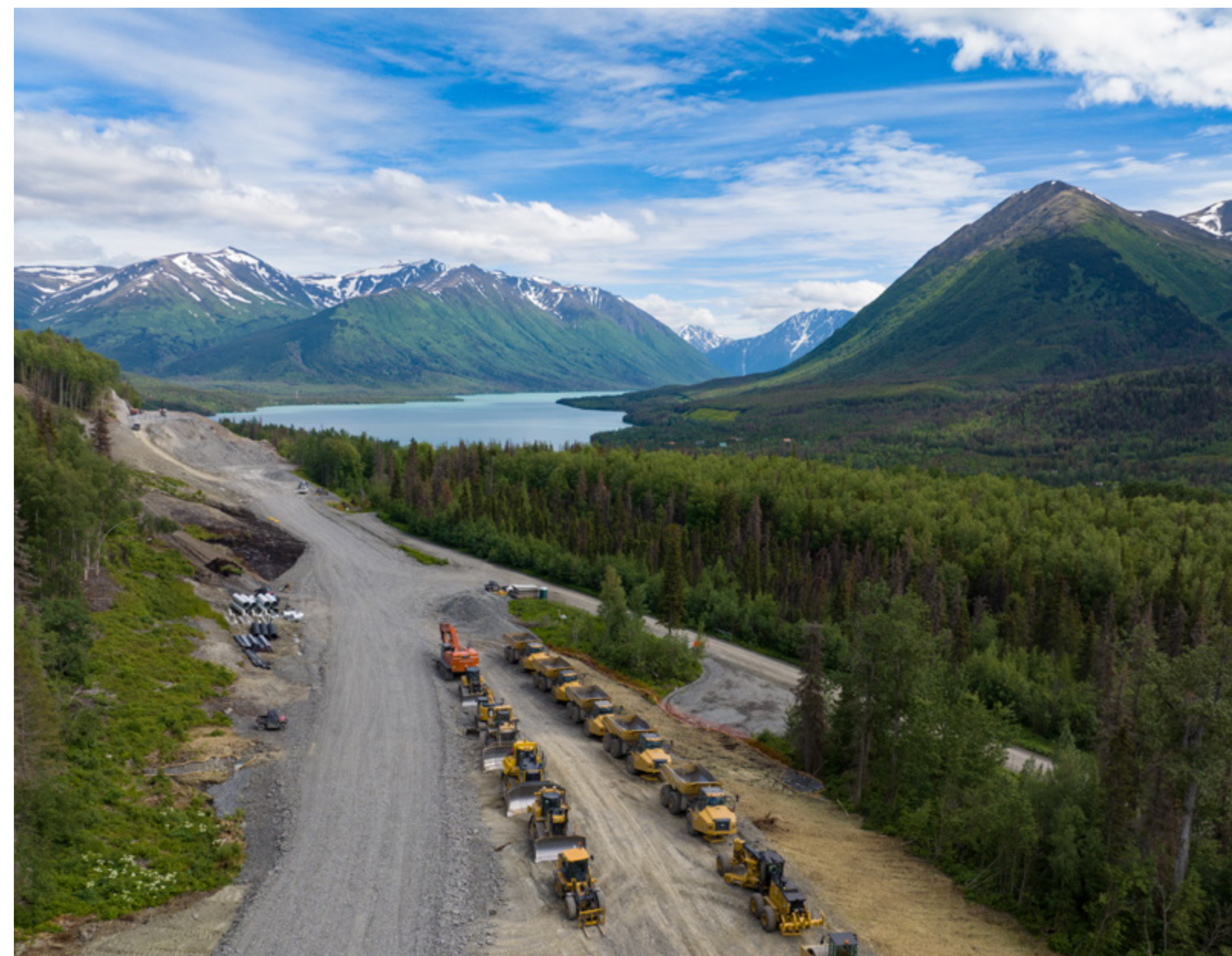
Phase 3: Equipment lined up at the end of Langille Rd.
