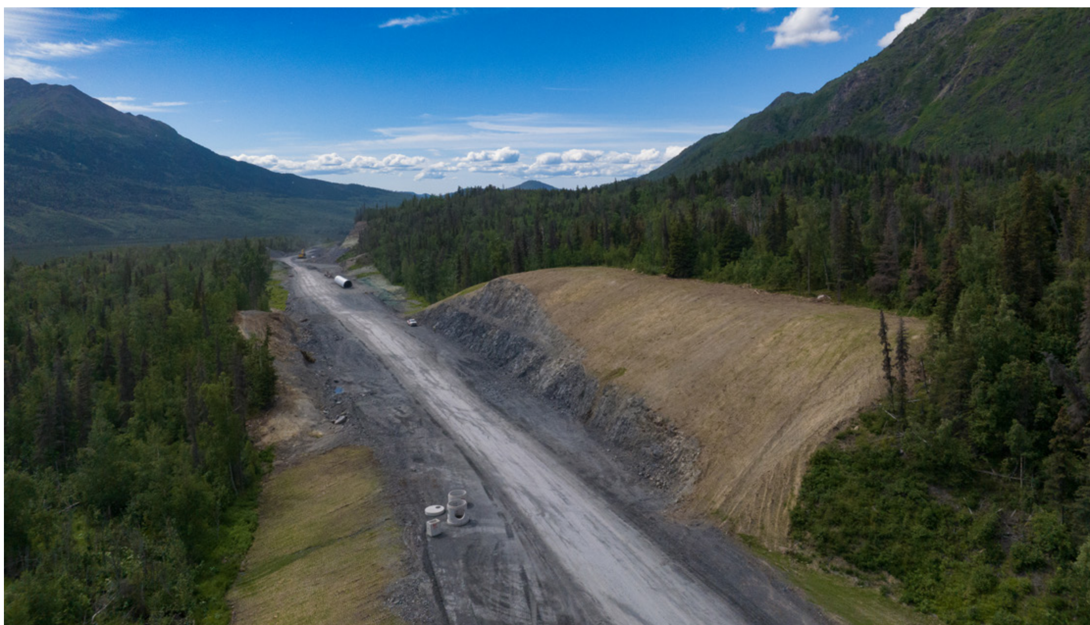
Blasting and Embankment is Mostly Complete
