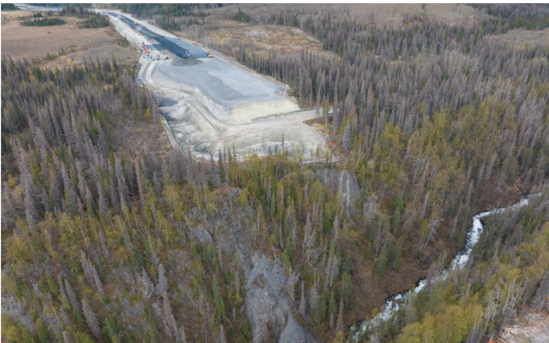
West Abutment: Excavation and Preparation for Pier Construction (2023)
