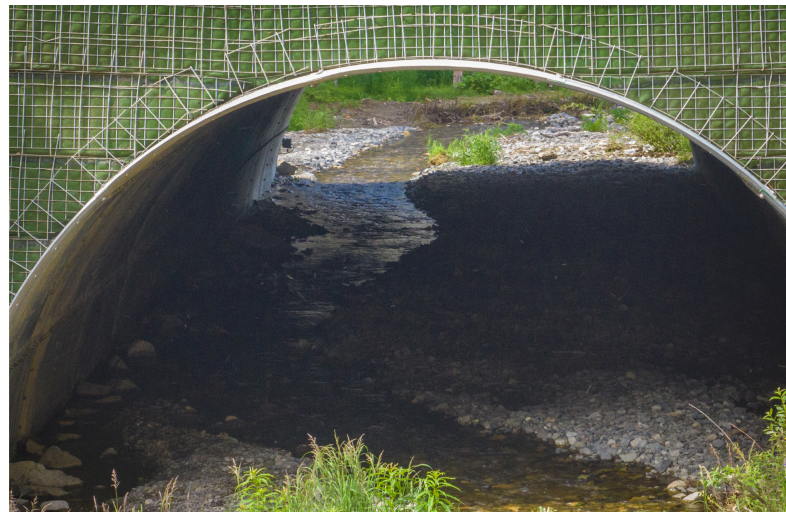
Inside Fuller Creek Wildlife and Fish Passage Crossing.
