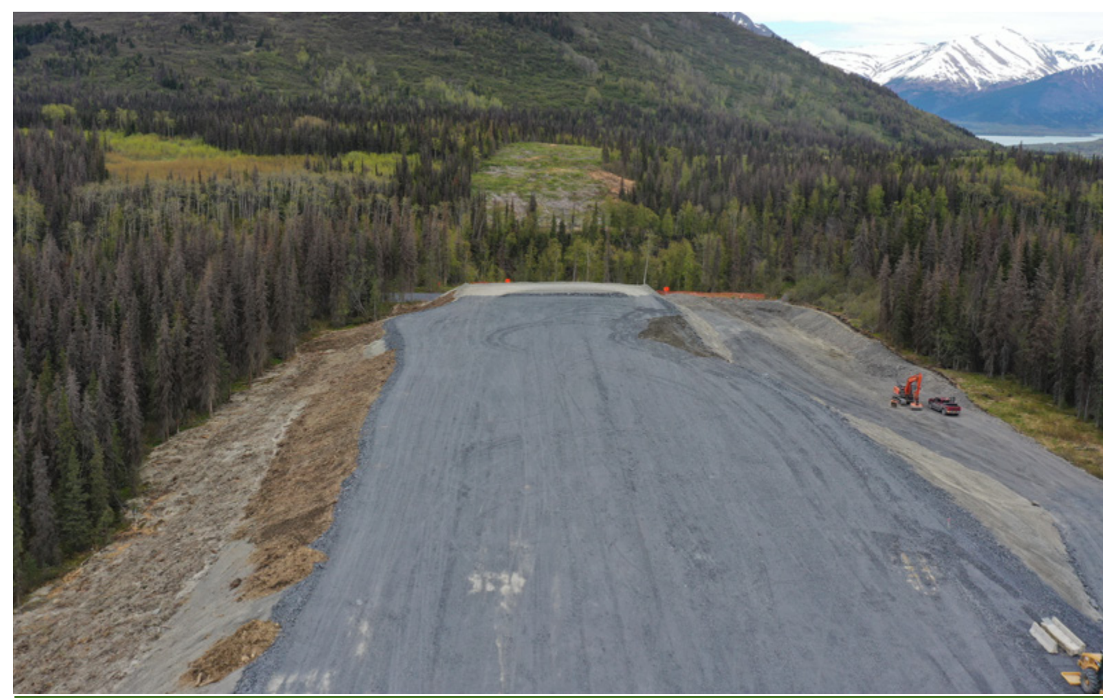
Phase 4: The West Bridge Abutment ready for equipment and materials.
