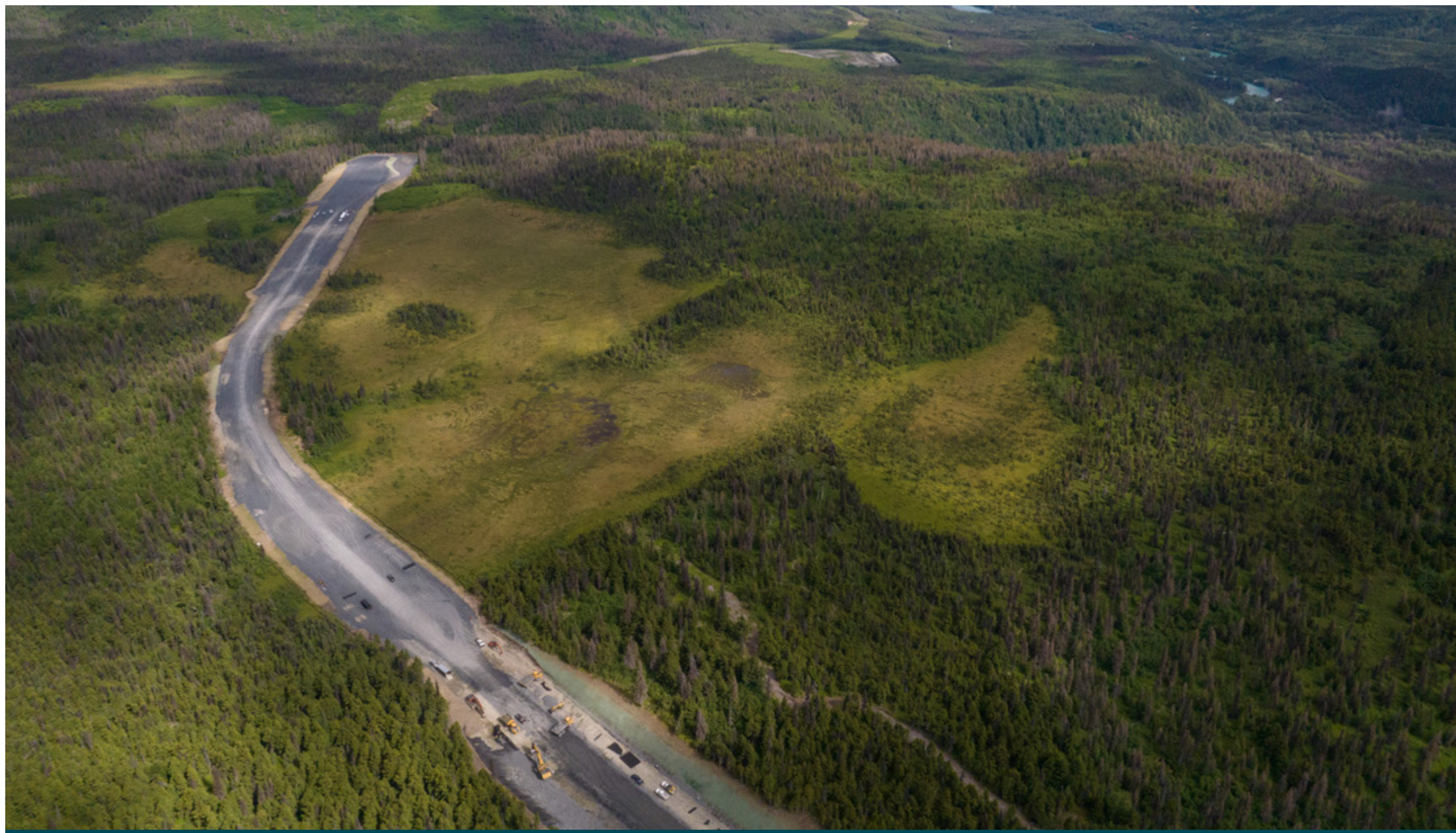
Access to West Abutment of Juneau Creek Bridge
