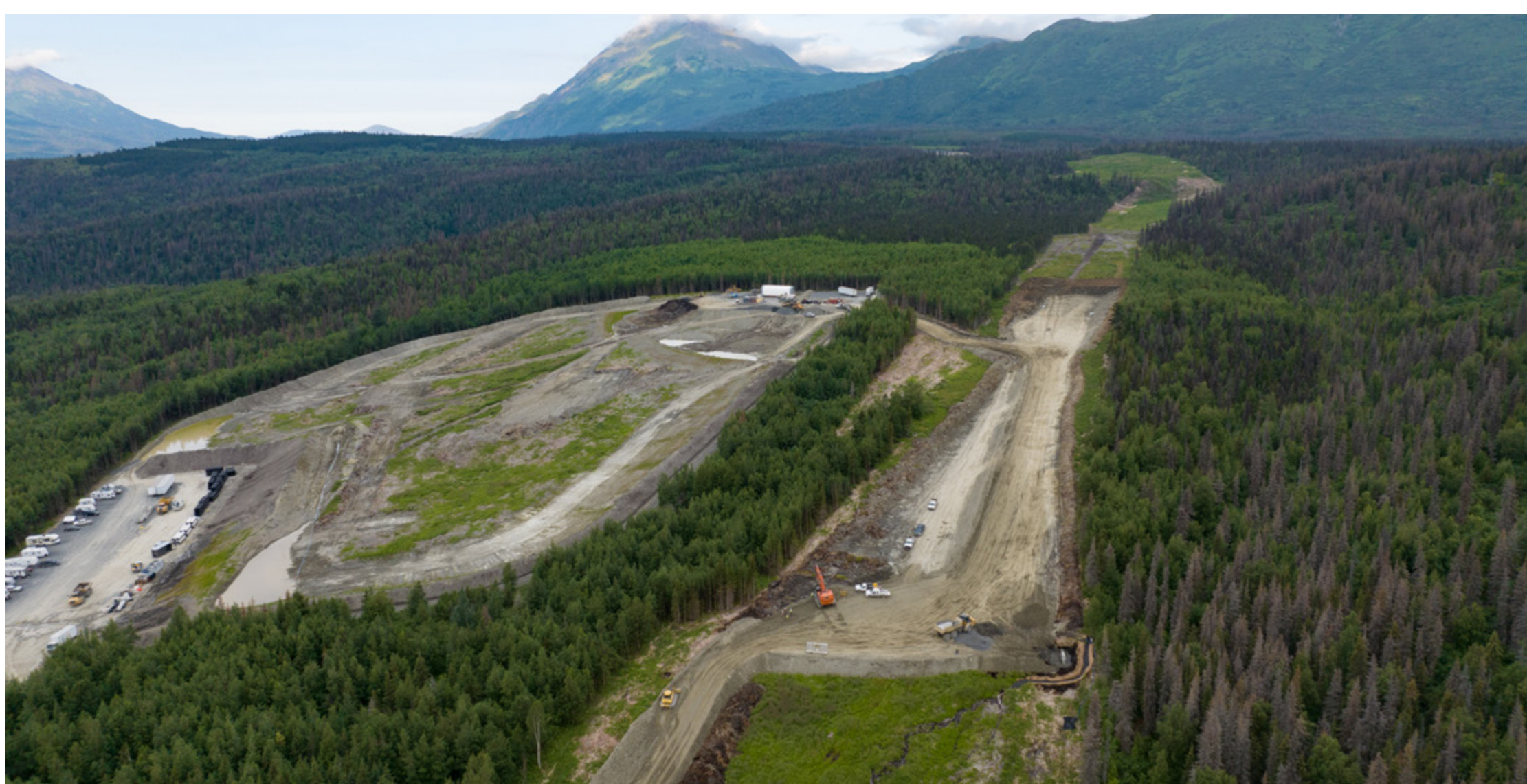
Access to Materials Disposal Site
